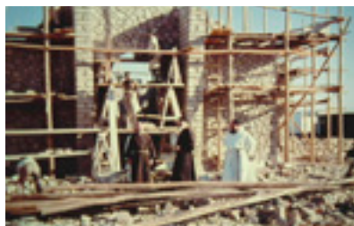
Active: Volunteers helping with the first DAHW project, the construction of a health station in Bisidimo
