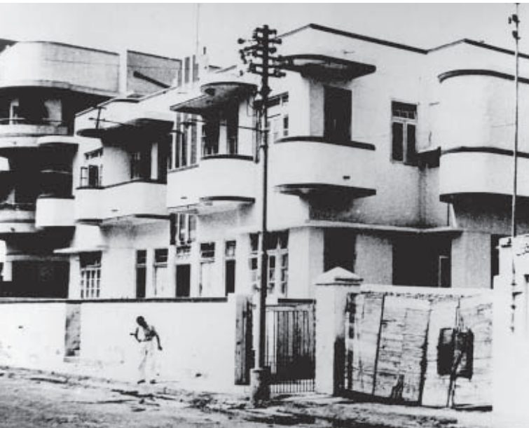
MALC-Krankenhaus in Karachi, Pakistan
